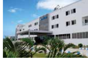
Rudrapur Plant (Green Building)
